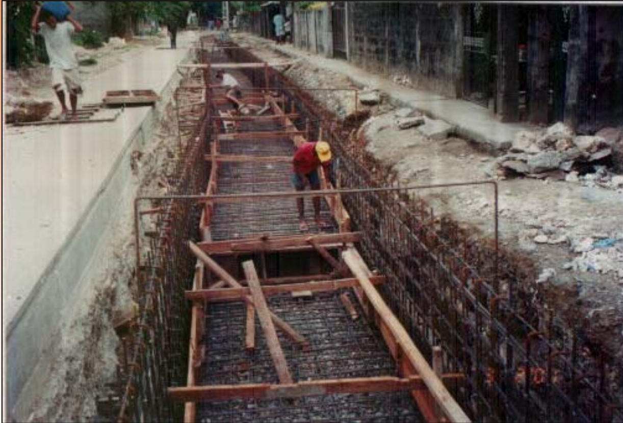
San Fernando City's Drainage Improvement Project
